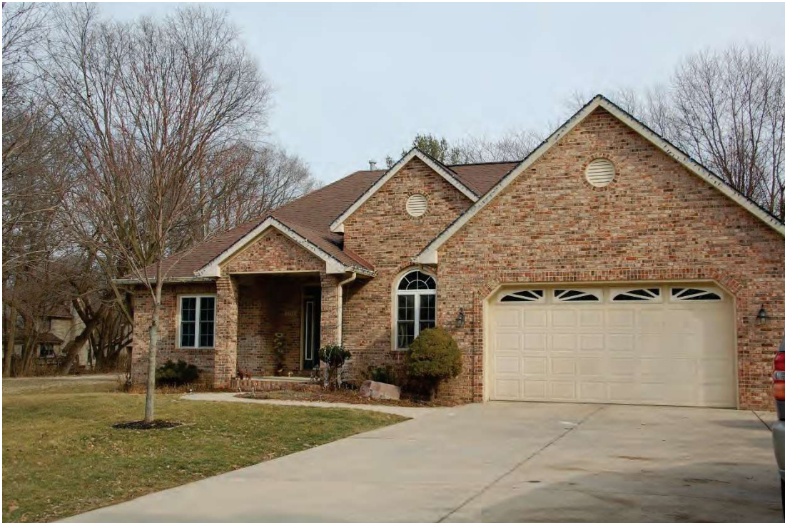
Photo 18. View looking northeast showing the façade of the house at 2710 Soldiers Home Road (ca. 2000)
