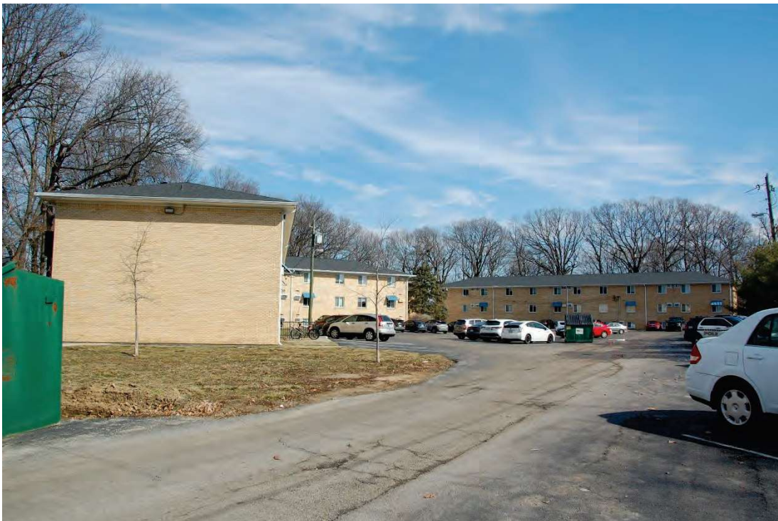
Photo 2. View looking northeast showing Happy Hollow Apartments, 2410 Happy Hollow Road (AL-001, ca. 1965, rated Contributing [C])
