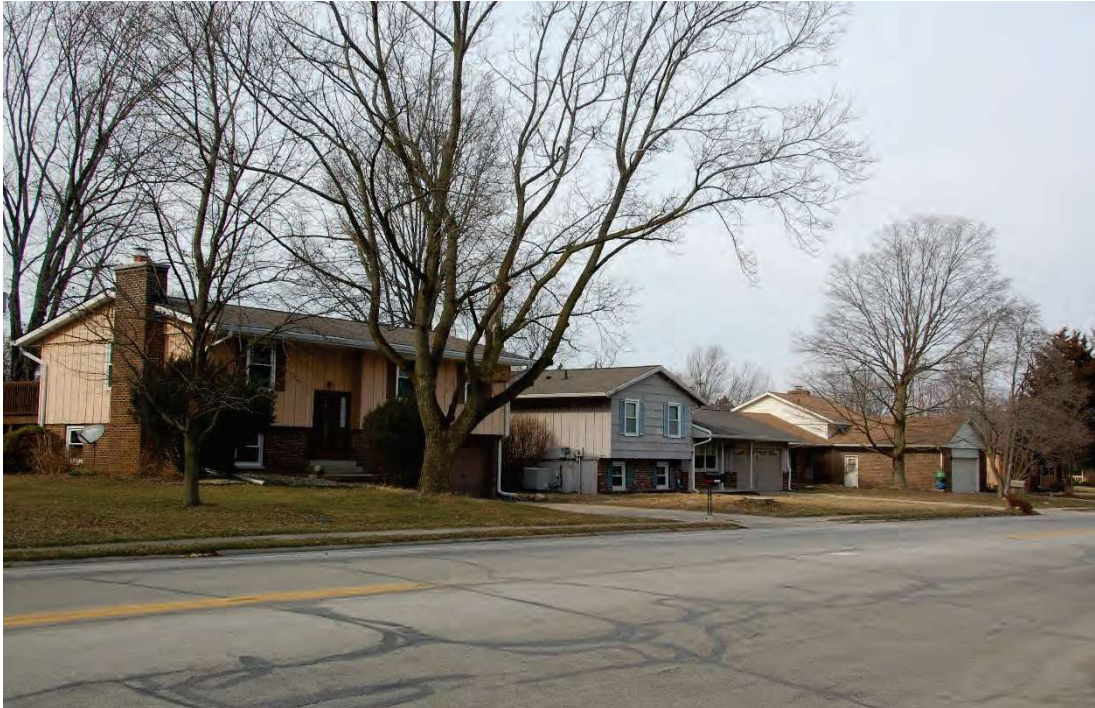
Photo 28. Streetscape view looking northwest showing houses at (left to right) 2955 Soldiers Home Road (AL-011, ca. 1976, rated C), 2963 Soldiers Home Road (AL-012, ca. 1978, rated C), and 2971 Soldiers Home Road (ca. 1978, rated NC due to alterations such as siding, doors, and an addition) from Soldiers Home Road
