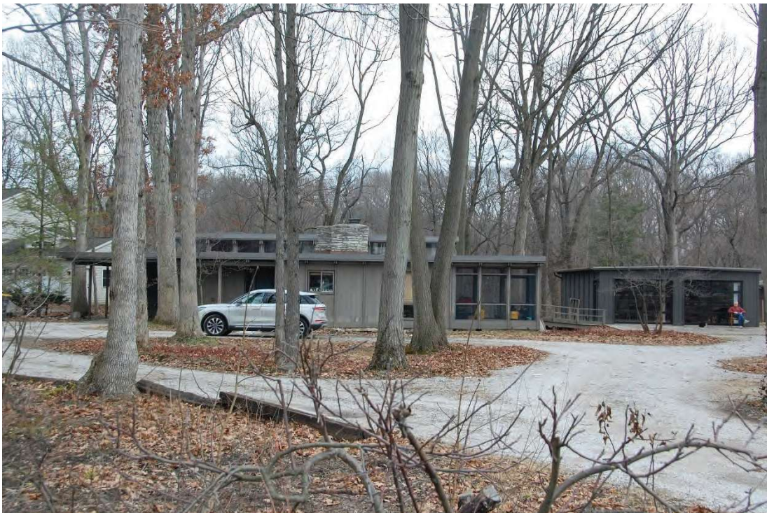
Photo 48. View looking east showing the façade of the house at 3211 Soldiers Home Road (AL-020, c.1961, rated Outstanding)
