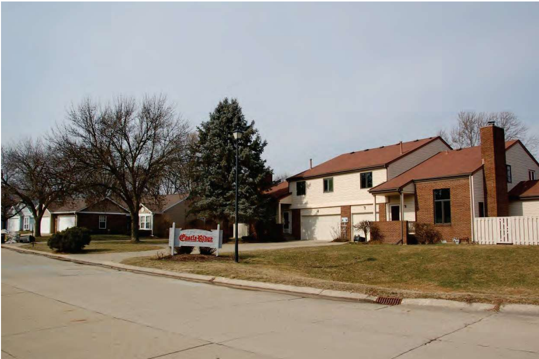
Photo 16. Streetscape view looking northwest showing 122-124 Westview Circle (ca. 1980) from the intersection of Westview Circle and Soldiers Home Road
