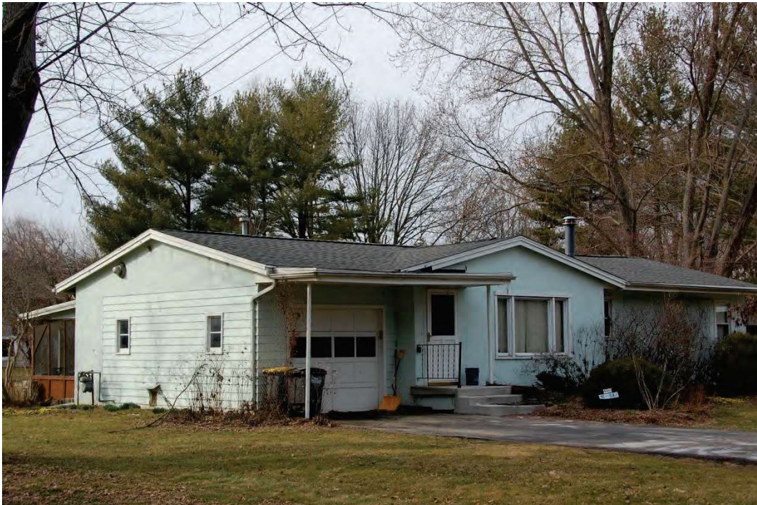
Photo 44. View looking northwest showing the façade and south elevation of 3142 Soldiers Home Road (AL-018, ca. 1957, rated C)
