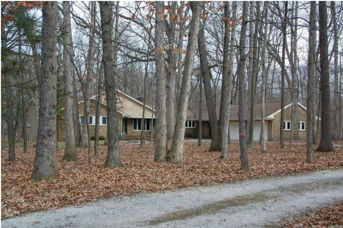
Photo 38. View looking southeast showing the façade of the house at 3011 Soldiers Home Road (AL-015, ca. 1950, rated C)
