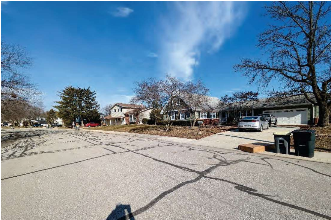
Photo 3. Streetscape view looking northwest showing (right to left) 132 – 116 Knox Drive within the Wabash Shores Historic District (AL-002, 1956-1973, recommended NRHP eligible) from Knox Drive
