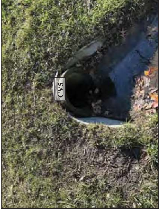
14. View of CV5 outlet, looking northeast.
