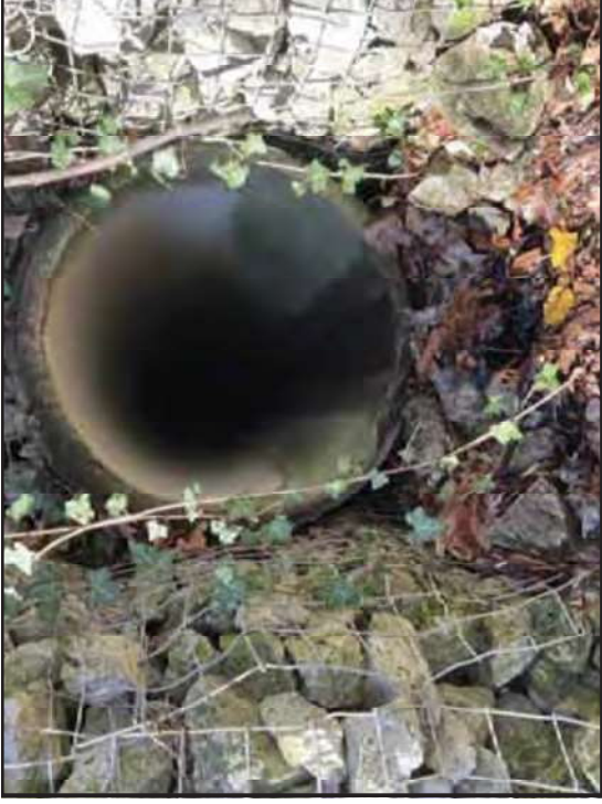
46. View of CV11 outlet, looking northwest.
